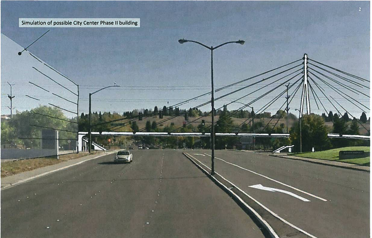
Illinger Canyon Road / Option 1-A – Cable-Stayed – Split (A-Frame) Main Tower/ South – looking east between Camino Ramon and Iron Horse Tra
