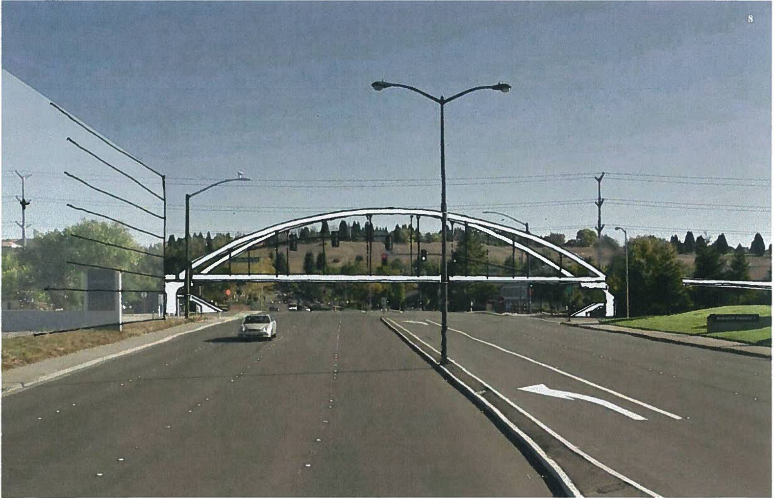
Illinger Canyon Road / Option 2 – Tied Arch – looking east between Camino Ramon and Iron Horse Trail
