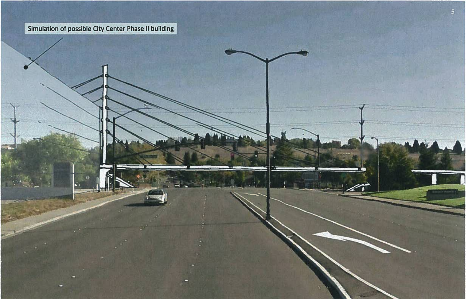
Illinger Canyon Road / Option 1-B – Cable-Stayed - Single Mast Main Tower / North – looking east between Camino Ramon and Iron Horse Trail
