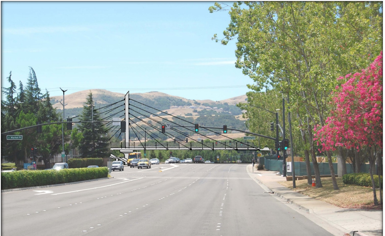
Bollinger Canyon Road / Option 1-A – Cable-Stayed – Single Mast Main Tower / South – looking west BCR Team
