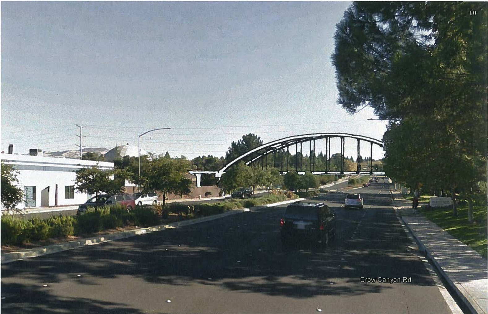
Crow Canyon Road / Option 1 – Tied Arch – looking east between Camino Ramon and Iron Horse Trail
