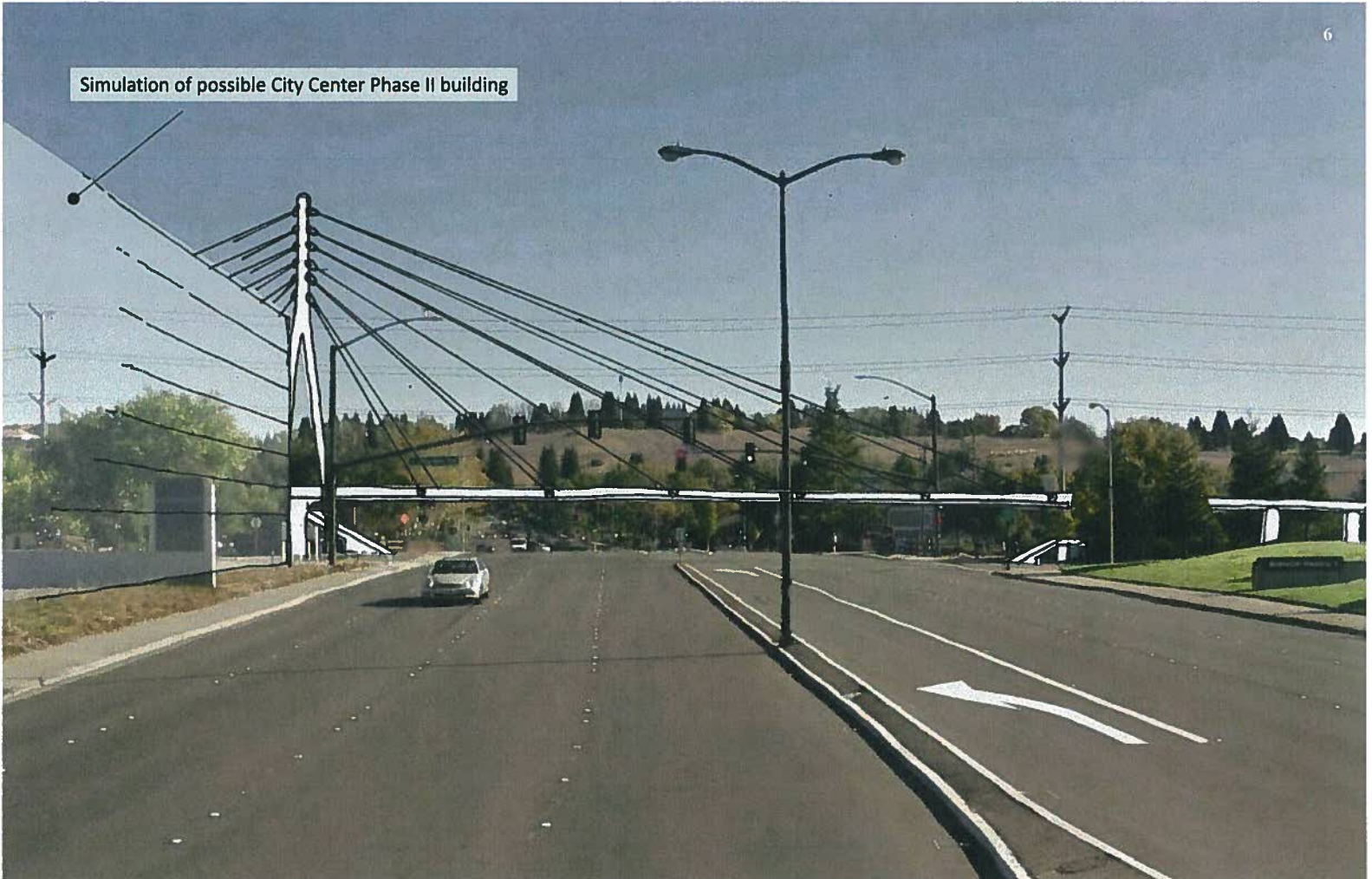
Illinger Canyon Road / Option 1-B – Cable-Stayed – Split (A-Frame) Main Tower / North – looking east between Camino Ramon and Iron Horse Tr
